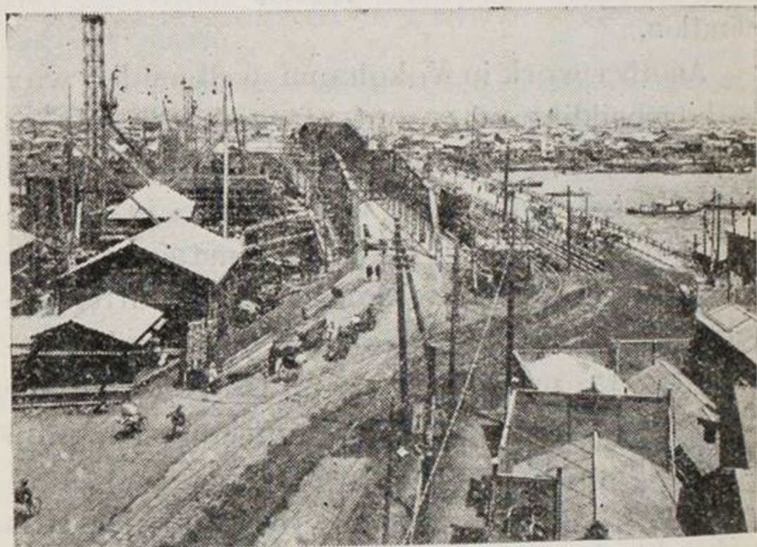
Reconstruction work in Tokyo, soon after the earthquake disaster.
